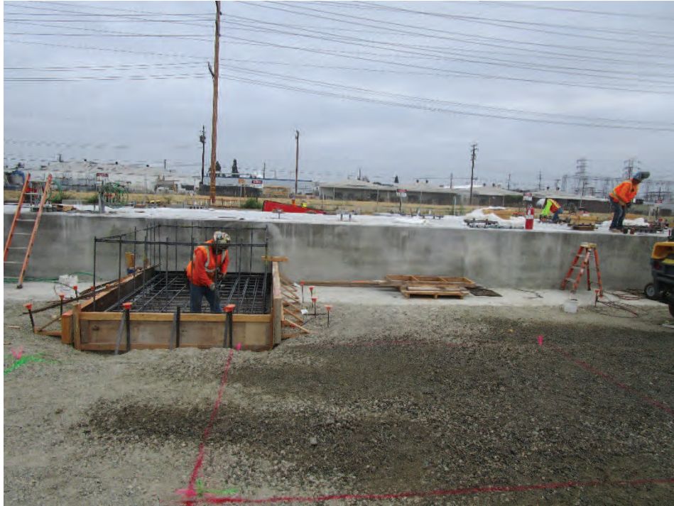
7/9/2019: U2 Oily Water Waste Tank Foundation Base Slab Formwork and Reinforcement
