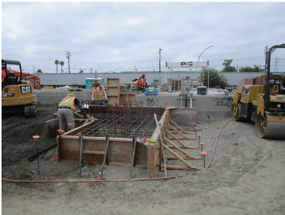
7/9/2019: Utility Rack Foundation Type 1 Formwork and Reinforcement
