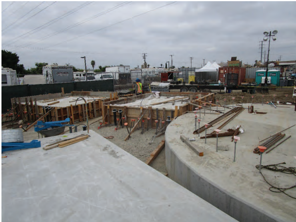
7/9/2019: Formwork Before Removal on Demin Water Skid and Fogging Water Recycle Tank Foundation
