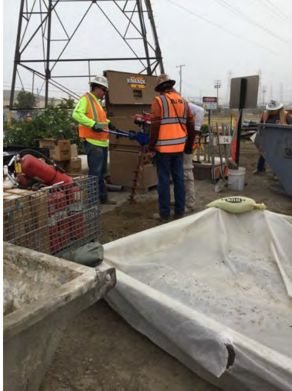
6in auger used to drill a 5' deep hole.
