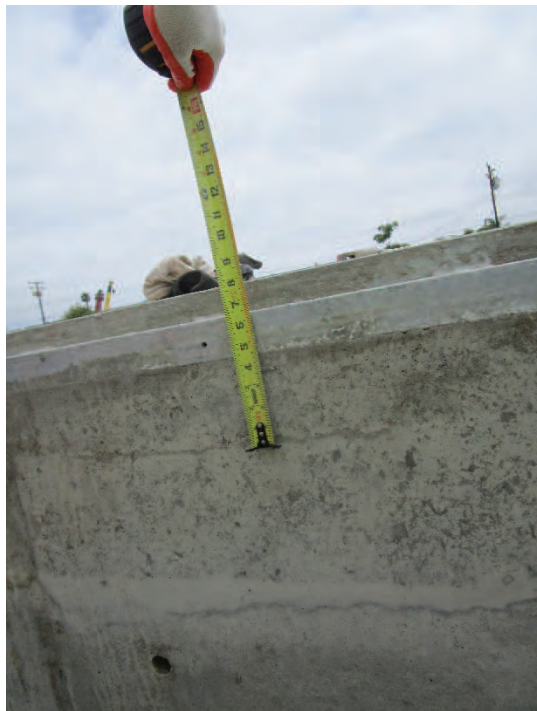
6/24/2019: GSU Pedestal Cold Joint Elevation Measurement 2
