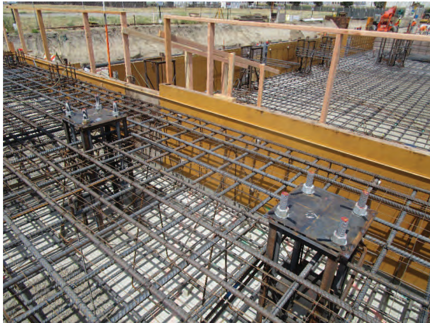
6/24/2019: CTG2 Foundation 02-MK1 Anchor Bolts in Foreground, ERU 2 Foundation Formwork and Reinforcement in Background
