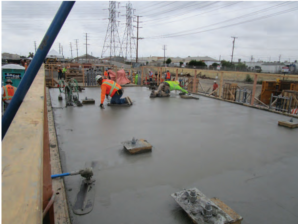
6/25/2019: CTG2 Concrete Surface Finishing
