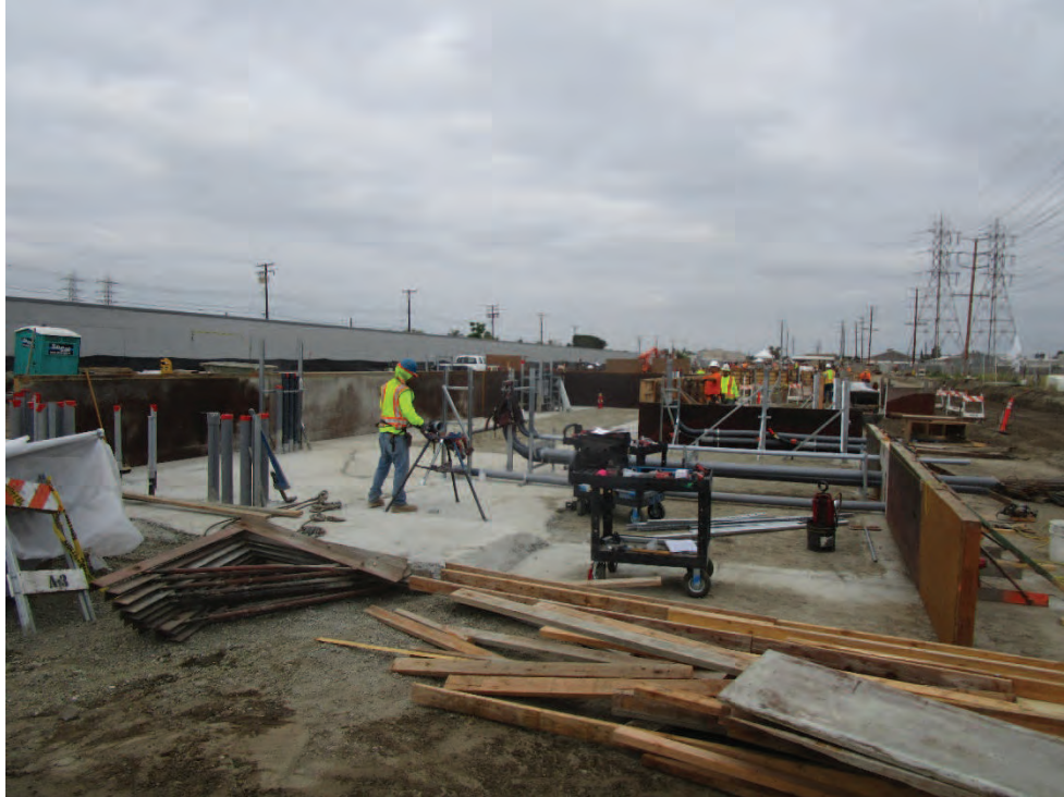
7/9/2019: CTG1 Formwork Assembly
