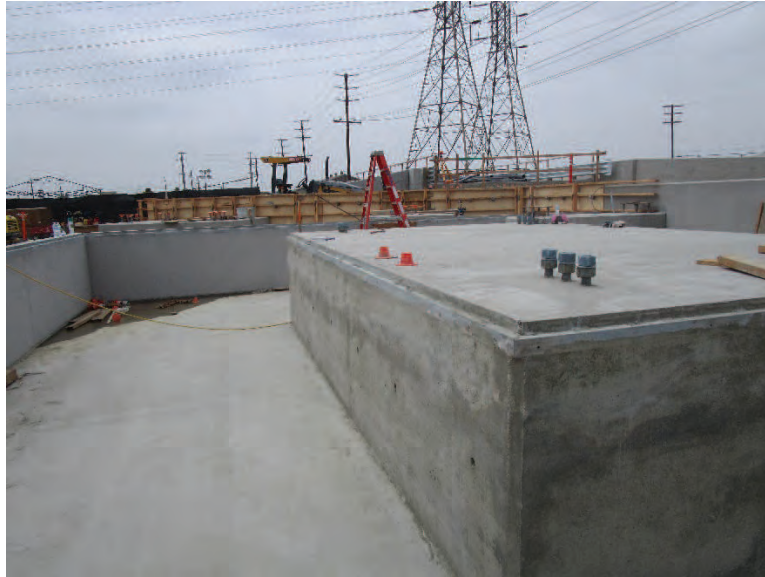
6/24/2019: GSU Pedestal Cold Joint – East Face
