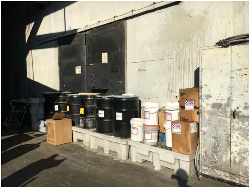
Photo 38: The site, facing northwest along the southern edge of mill building loading dock, with additional hazardous materials/waste drums (including universal wastes) on plastic secondary containment.
