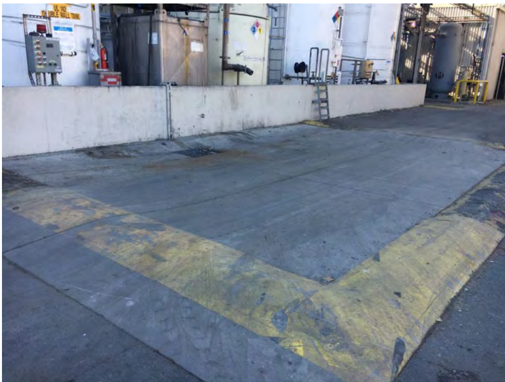
Photo 20: The site, facing southwest towards the wet end tank farm unloading area within bermed pad with bottom sump (water pumped back into mill reservoirs).
