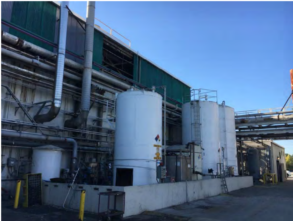
Photo 19: The site, facing southwest towards the wet end chemical storage tank farm at mill northwest corner, with 4,000 to 20,000 gallon tanks for bulk storage of water treatment chemicals, within berm containment.
