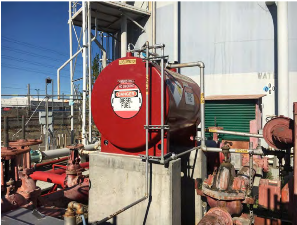
Photo 8: The site, facing northwest towards 300 gallon diesel AST above bermed containment, south of water AST.
