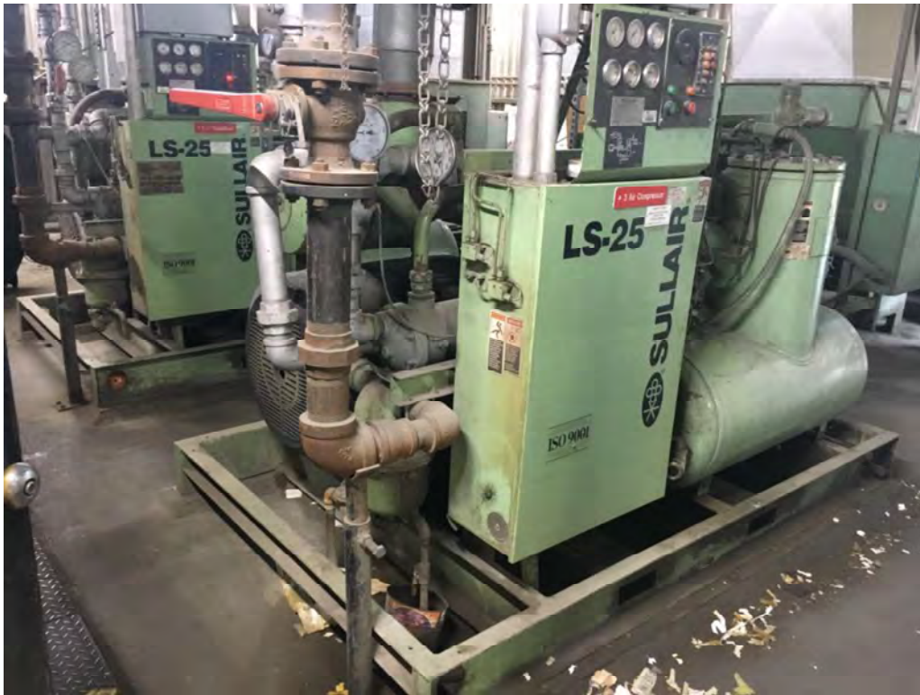
Photo 27: The site, facing east towards air compressors within the air compressor shed, with drip pans on far underside of units.
