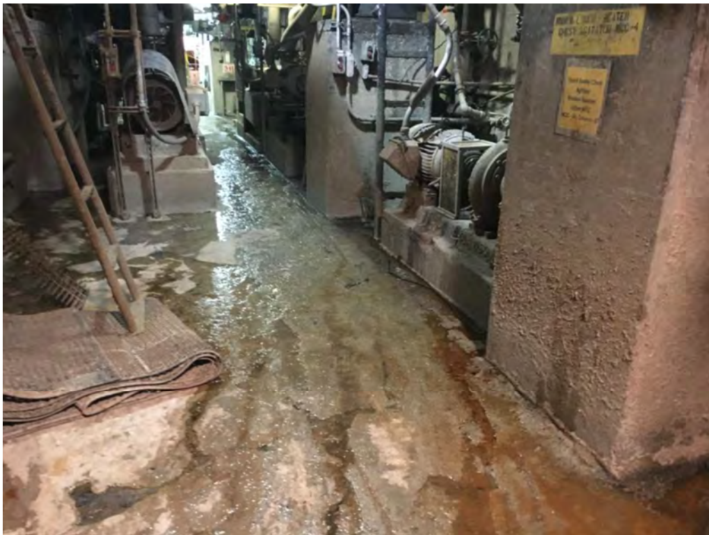
Photo 56: The site, facing northwest within the below-ground basement area. Groundwater intrusion is visible in this area.
