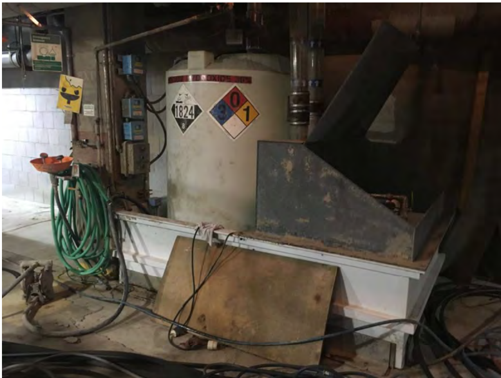
Photo 58: The site, facing northwest within the below-ground basement area. A 400 gallon aboveground container is located here within secondary containment for sodium hydroxide, conveyed here from the northwestern exterior tank farm.
