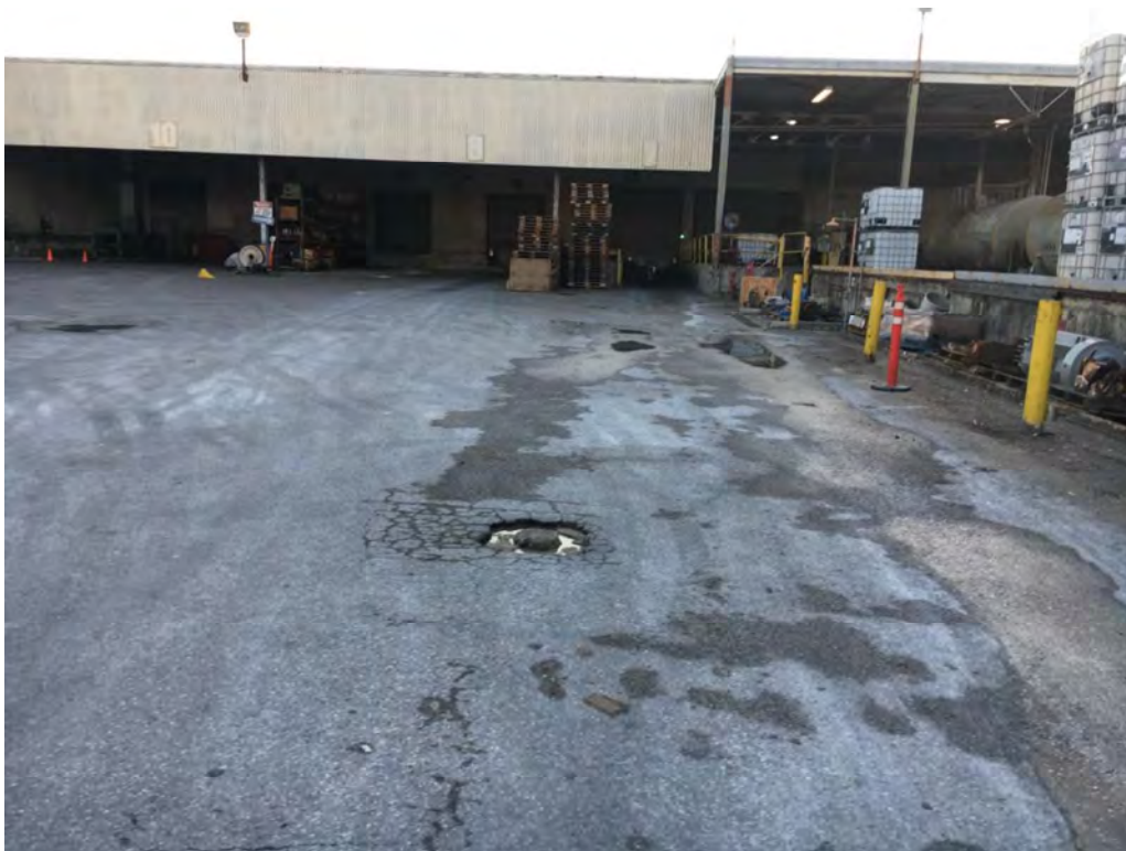
Photo 42: The site, facing east towards southeastern corner of central courtyard area. Abandoned former monitoring well locations are visible at center and beyond: the locations of former solvent and diesel USTs. A former gasoline UST is closed in place here.
