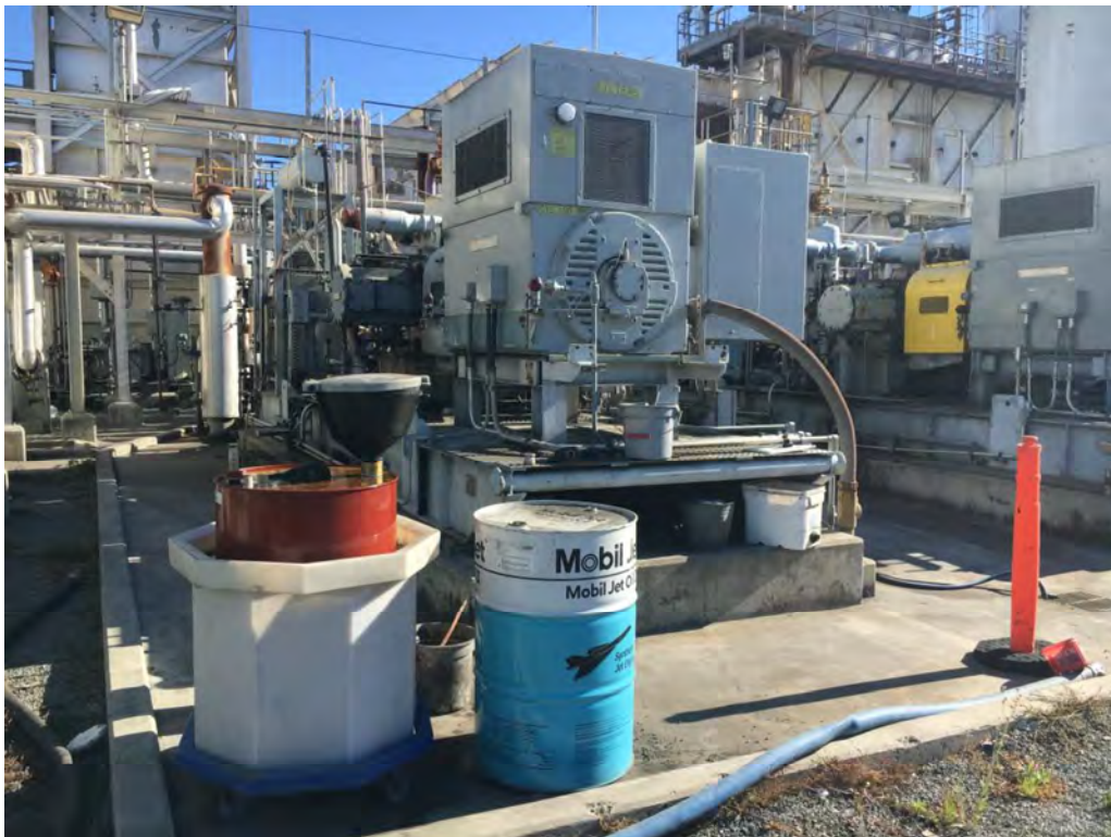
Photo 16: The site, facing east towards the northwestern corner of the cogeneration plant. Generators with gas compressor and petroleum product (jet fuel/petroleum) secondary containment are visible at center.
