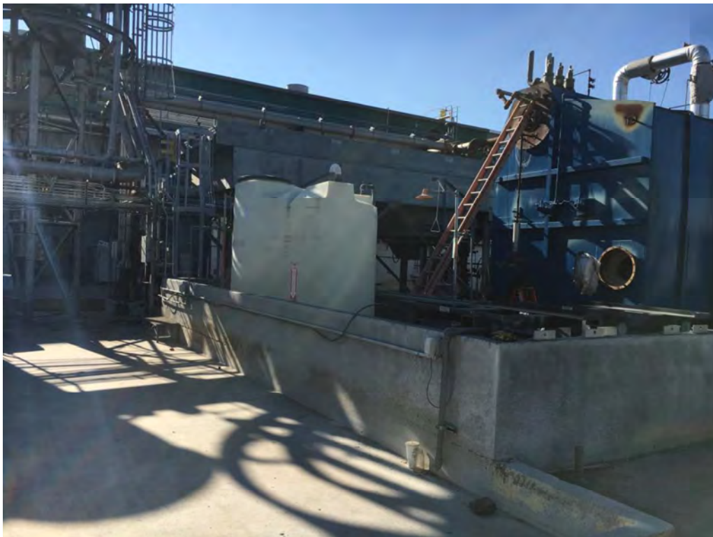
Photo 18: The site, facing south towards the northeastern cogeneration plant chemical storage area #2 within concrete bermed containment.
