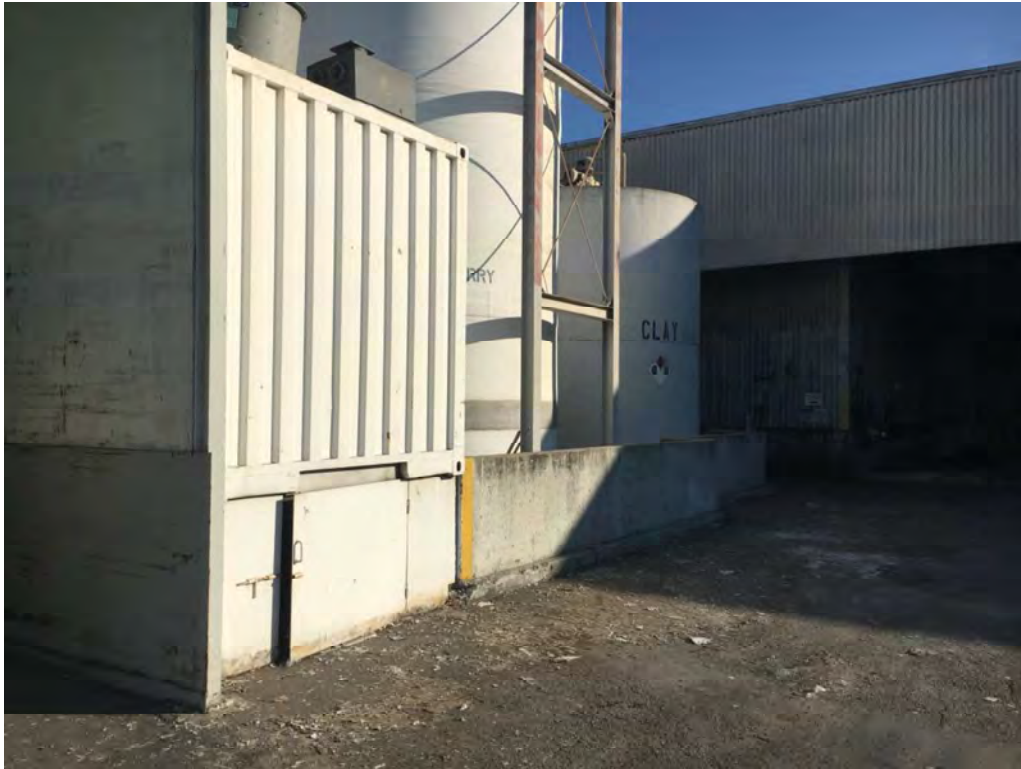
Photo 39: The site, facing northeast towards the coating bulk (clay) storage tank farm within concrete bermed secondary containment.
