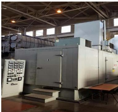
Vernon owns and operates two natural gas-fired combustion turbine units (H. Gonzales Generating Station #1 and #2), which are also located within the City of Vernon. The H. Gonzales natural gas-fueled combustion turbines are Allison 571-KA combustion turbines, rated at 5.75 MW each. The combustion turbine units began commercial operation in 1988. Each of the units is restricted by air quality regulators to run on natural gas for no more than six hours per day.
