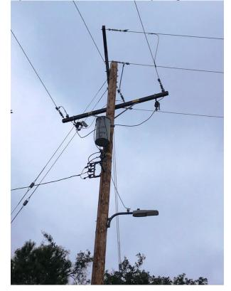
Figure 44: Example of Increased Conductor Spacing in LADWP Territory
