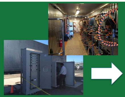
500 kWh Prototype "Grid-Saver" system (CEC-funded, 2011-2014)
