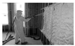
Figure 3-20: Open-Cell SPF Installed in Wall Cavity
