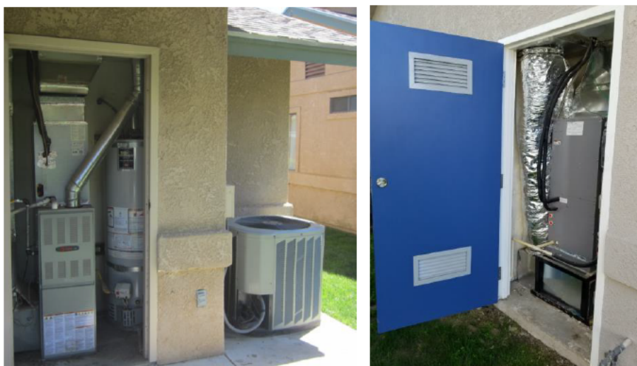
Existing Gas Furnace (left), New Heat Pump HVAC (right)
