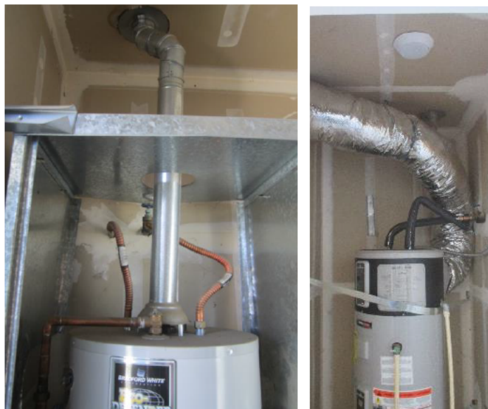
Existing Gas Water Heaters (left), New Heat Pump Water Heater (right)
