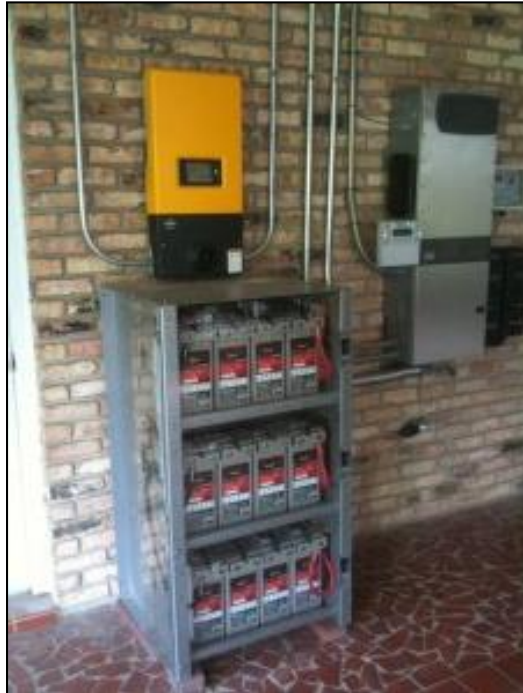
Figure C-12 An Outback Power installation with lead-acid batteries.
