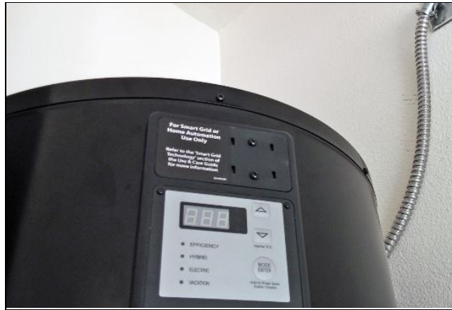
Figure 4-8 Communications port provided by water heater
