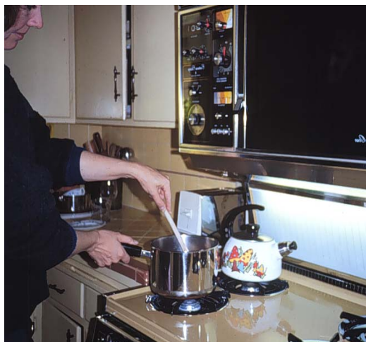
Unvented appliances are sources of nitrogen dioxide, carbon monoxide, and other pollutants.
