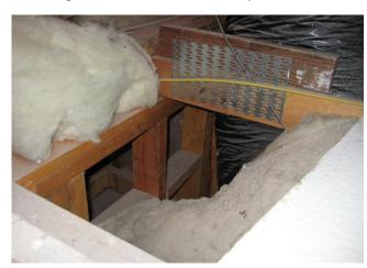
Figure 60: Leakage between Conditioned Space and Attic
