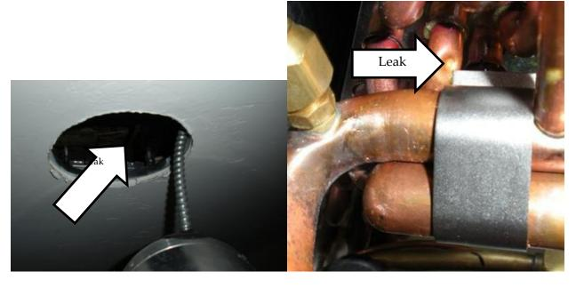
One leak is accessible through a recessed lamp, the other from the TXV bulb clip. Photo Credit: Rick Chitwood
