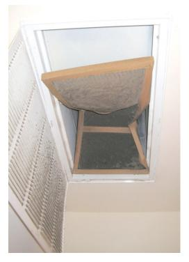
This 14 in. X 30 in. X 1 in. standard filter is so dirty it is sucked into the return duct that is substantially smaller than the return grille. The home owner is sufficiently embarrassed that he offers to go to the store and bring back a new filter. He is instructed specifically to bring back a low efficiency, low cost filter.
