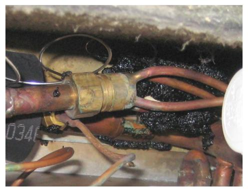
Figure 19: Unit 58—Melted TXV Bulb Insulation
