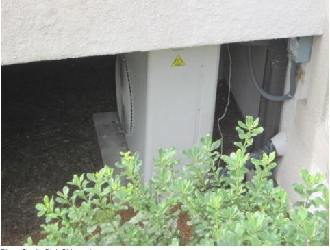
Figure 20: Unit 72—Condenser Recirculation
