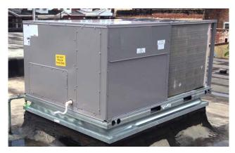
Figure 3: Illustration of a packaged rooftop air conditioning unit
