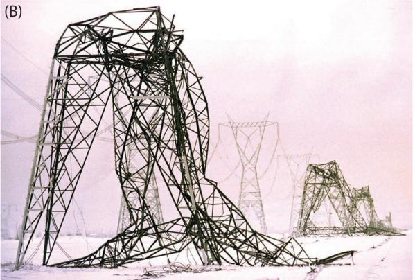
FIGURE 3.10 (A) Ice accumulation of several inches on distribution lines caused these poles to collapse, and (B) images from the infamous 1998 ice storm across southeastern Canada and the northeastern United States.
