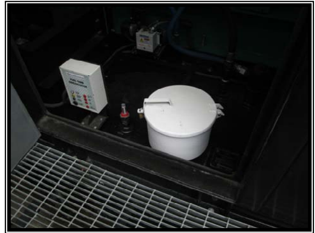
PHOTO 4: Diesel overflow /spill bucket in older backup generator unit.
