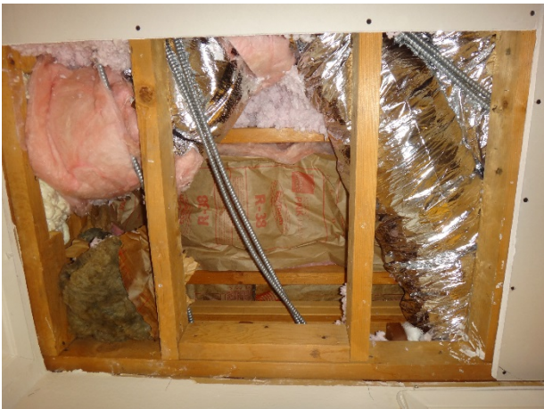
Old and new ductwork
