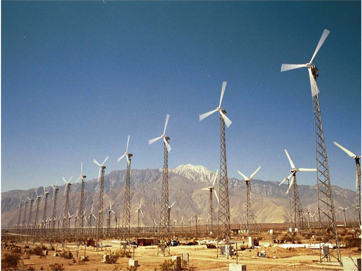
Figure 10. AASI's windplant of 13, 50 kW nameplate, downwind, free-yaw turbines in A-row, at 62450 Dillon Rd, North Palm Springs, CA 92258. This windplant of vintage-1985 turbines delivered electricity to the SCE grid from 1991- 2012, when the PPA expired. AASI intends to reconfigure this windplant to deliver 100 % of its captured energy as Hydrogen transportation fuel, with no connection to the grid, for fuel cell cars, buses, trucks. Hydrogen delivery will be via tube trailer in the short term, then via a new, dedicated, high-purity, underground Hydrogen pipeline system for gathering and transmission, firming storage, and distribution. An attractive Hydrogen fuel customer is Sunline Transit, 15 miles east on I-10, at Thousand Palms, which operates fuel cell buses.
