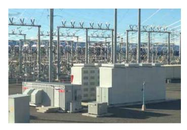
The sodium sulfur battery located at the Pacific Gas and Electric facility in Vaca-Dixon, CA was the first to provide services to the ISO market. Utility scale energy storage such as this one offers significant flexibility in balancing the grid under a variety of conditions. The potential operational benefits include:
