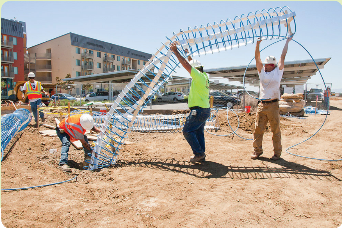
Figure ES-3: Low-Cost Ground-Coupled Heat Pumps being Installed Source: California Energy Commission, Energy Innovation Showcase
