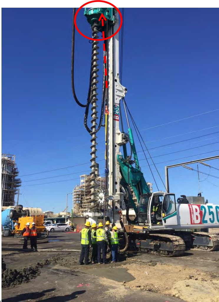
Center bar contacted rotary head while being positioned for placement in hole.
