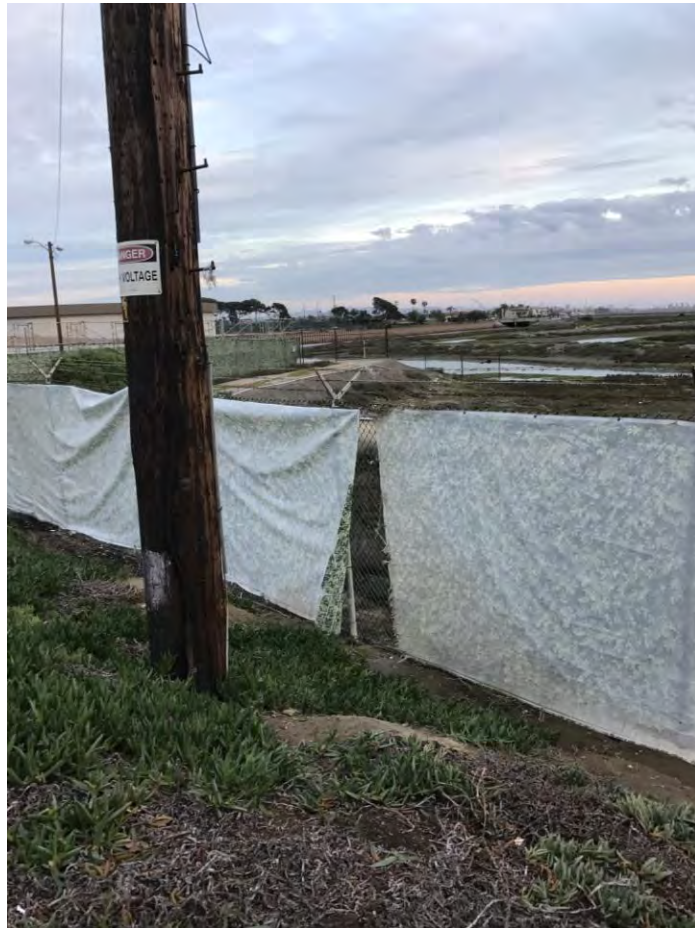
Damaged Construction Screening
