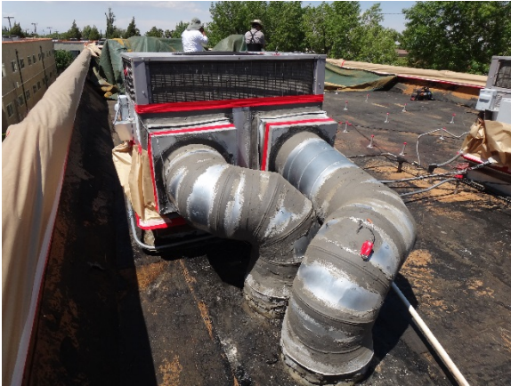
Old and new ductwork
