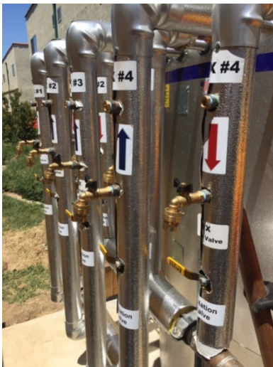
Solar Thermal Heat Exchanger Piping
