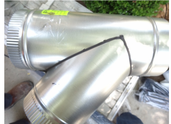
New duct joints
