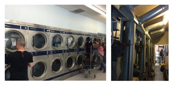
Figure 5.2 Laundromat dryer installation. Left: dryers installed parallel to exterior wall, Right: unconditioned service access area between wall of dryers and exterior wall
