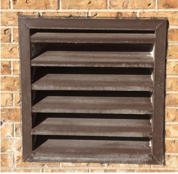
**Figure 5.3 Example of wall grate in service area enabling outdoor air flow to dryer intake (photo taken from exterior of building)**
