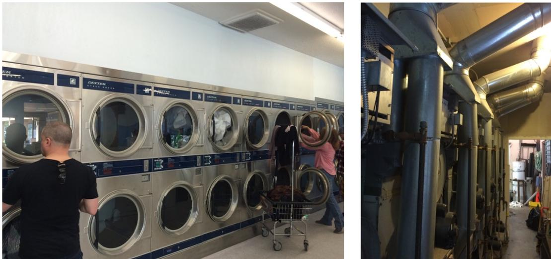
**Figure 5.2 Laundromat dryer installation. Left: dryers installed parallel to exterior wall, Right: unconditioned service access area between wall of dryers and exterior wall**
