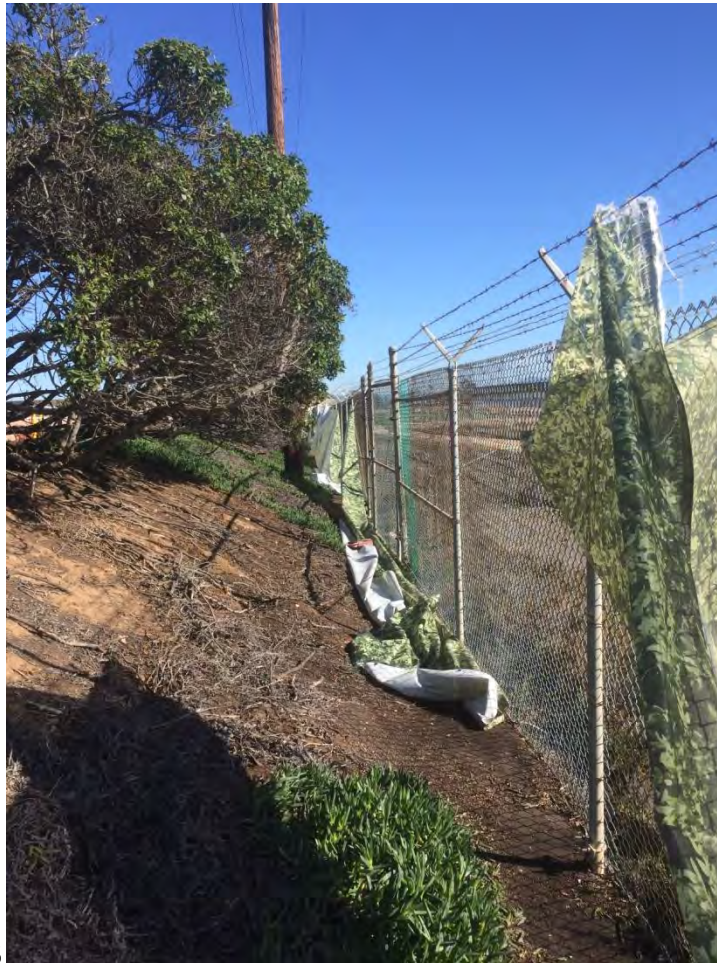
Damaged Construction Screening
