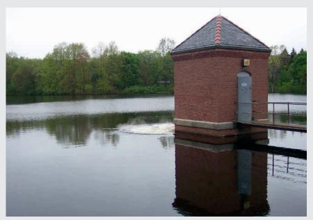
The process flushes the debris away from the screen surface by releasing a large volume of compressed air through the bottom of the screen within a few seconds. The typical backwash procedure cleans each water intake either sequentially or at regular intervals.
