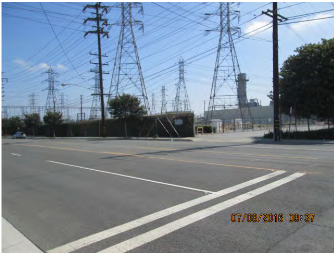
27. View of eastern adjacent Dale Avenue with the Barre Substation and Peaker Plant (10670 Dale Avenue) beyond, looking to the northeast.
