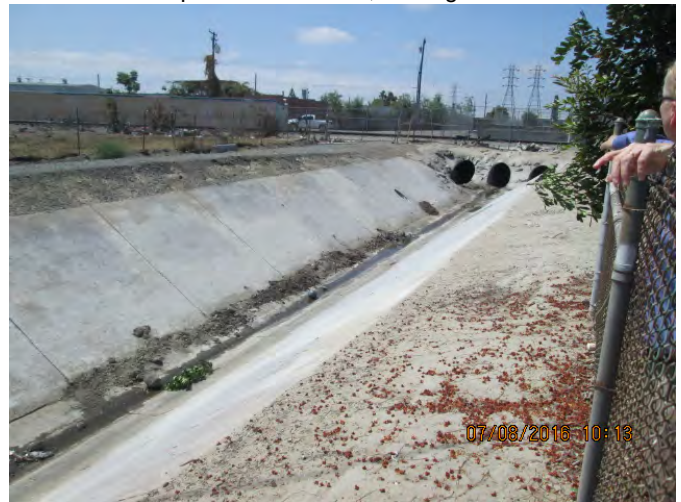
10. View of the central Stanton Storm Channel portion of the Site, looking to the southeast.
