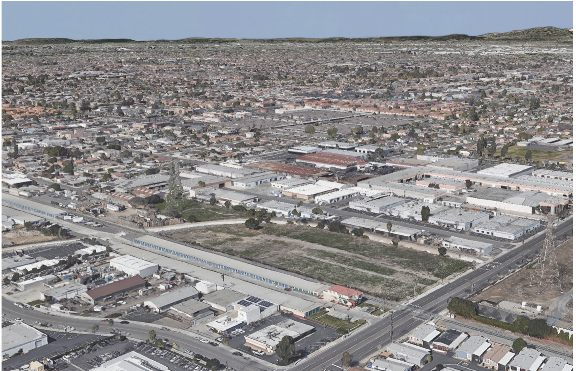
Figure 1.0-1 Project Site Prior to Construction Stanton Energy Reliability Center AFC Stanton, California
