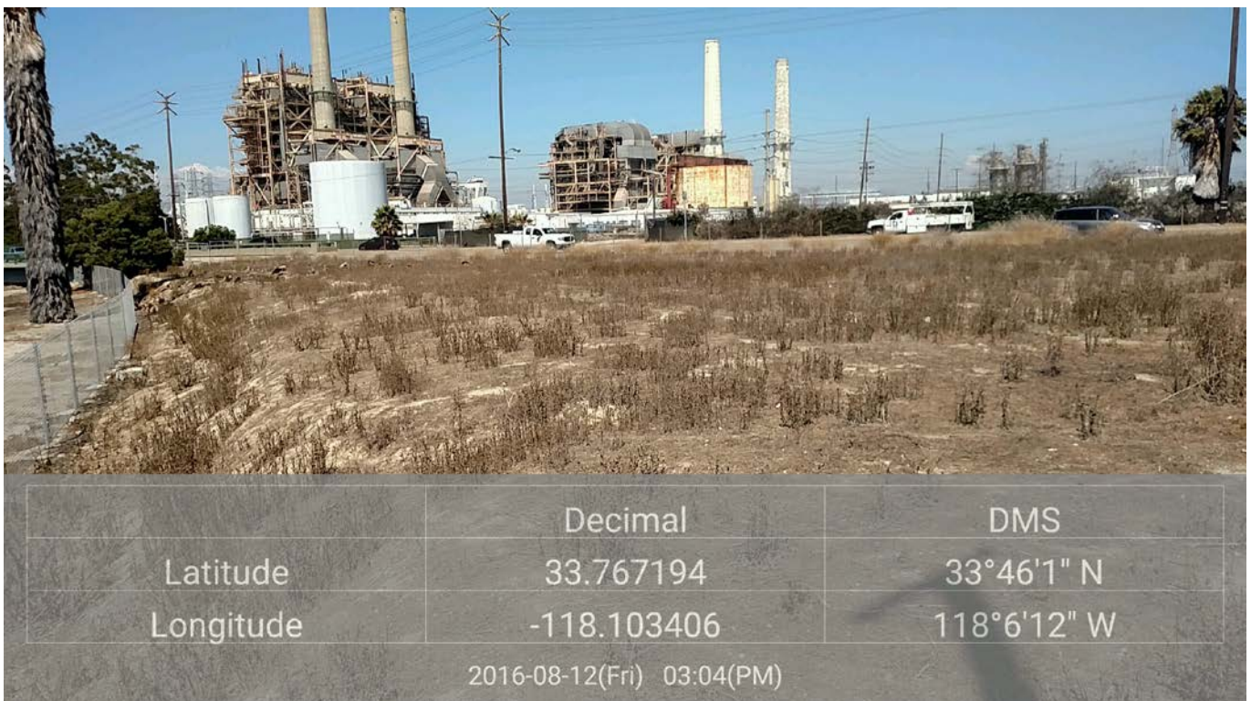
Photograph 6. Overview of the Survey Area associated with the proposed process and sanitary wastewater pipeline.
