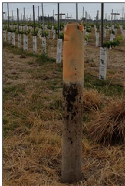
2 year old well (drilled 2010). Land surface shows 2 feet of subsidence (well location shown on map). Photo courtesy Sarge Green, California Water Institute.
