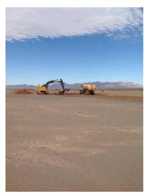
Photo 9: AQ SC-3: Construction Fugitive Dust Control
