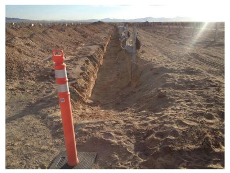
**Photo 3: Bio-2, Bio-4, Bio-8: Wildlife Entrapment** Trench ramped with a 3:1 slope for wildlife exit in Unit 1; November 10, 2015
