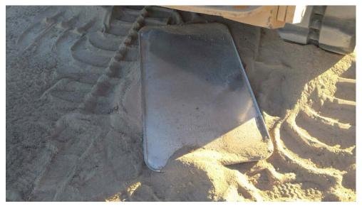
**Photo 2: Bio-8: Minimize Spills of Hazardous Materials** Drip pan in place beneath staged construction equipment; November 6, 2015
