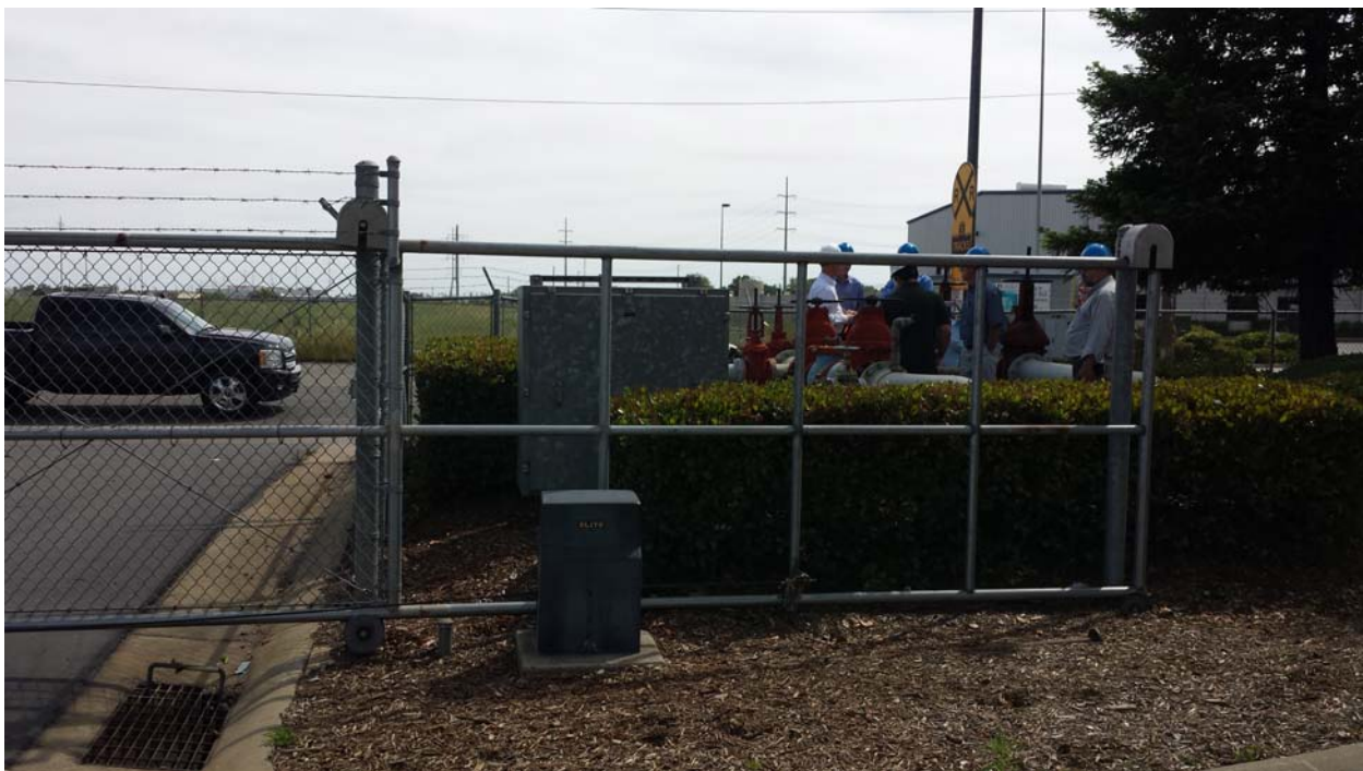
Photo 2. Western side of east entrance (shown in Photo 1), where the recycled water could be brought into the project from Regional San alongside the existing water service lines.
