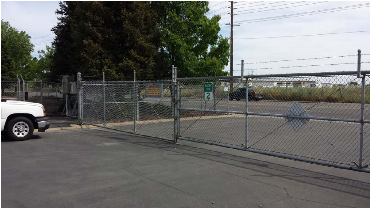
Photo 3. Entrance (shown in Photo 1). An option is being considered to place the recycled water line in an underground vault in the middle of this driveway.
