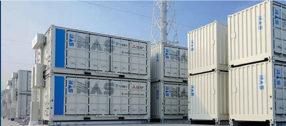
Kyushu Electric Power Co., Inc.'s new 300,000-kilowatt-hour NAS storage array, supplied by NGK Insulators, Ltd., helps balance supply and demand amid Kyushu's surging growth in solar generation. (NAS photo courtesy of Kyushu Electric)
