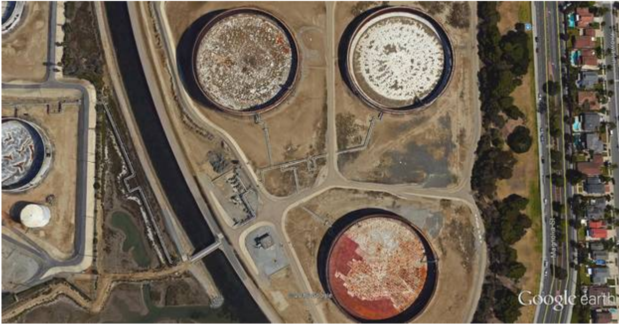
The screen image above is from Google Earth dated March 2015
