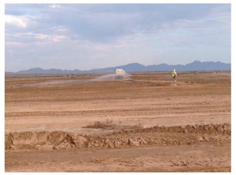
Photo 6: AQ SC-3: Construction Fugitive Dust Control Water was applied for dust control in Unit 2; October 12, 2015
