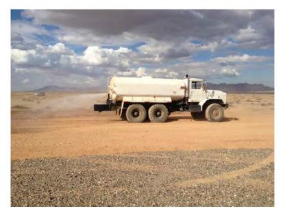
**Photo 3: AQ SC-3: Construction Fugitive Dust Control** Water was applied for dust control in Unit 2; October 5, 2015
