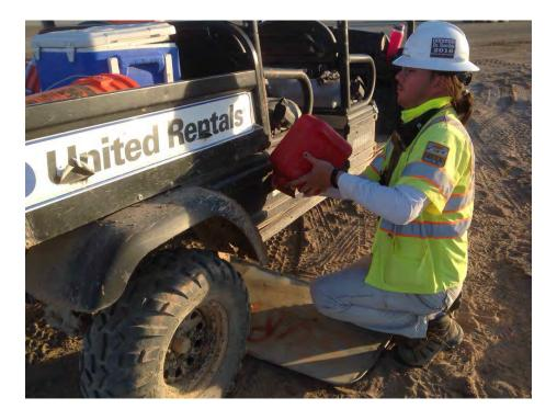
Photo 9: DF Bio-8: Minimize Spills of Hazardous Materials Control Drip pan being used while fueling a buggie in Unit 2; October 27, 2015
