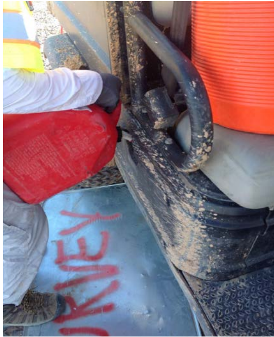
Photo 9: DF Bio-8: Minimize Spills of Hazardous Materials Control Refueling of cart with drip pan in place in Unit 2; September 24, 2015
