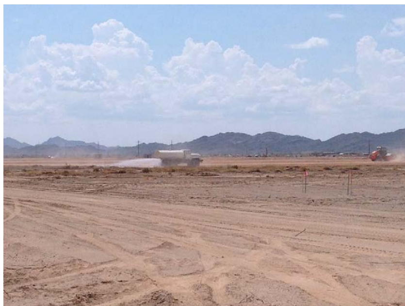
Photo 3: AQ SC-3: Construction Fugitive Dust Control Water truck watering work area in Unit 1; September 8, 2015
