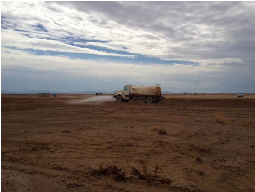
Photo 8: AQ SC-3: Construction Fugitive Dust Control Water was applied for dust control without causing ponding in Unit 1; September 21, 2015
