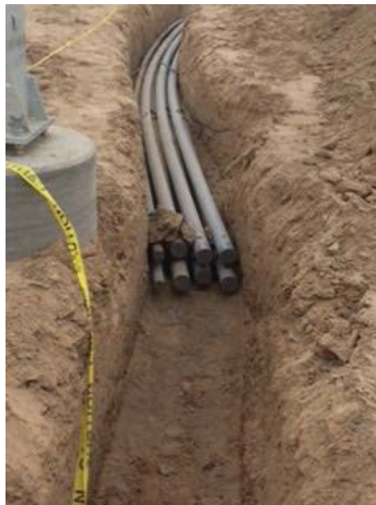
Photo 10: Bio-2, Bio-4, Bio-8: Wildlife Entrapment Conduit taped off to prevent wildlife entry in Unit 1; September 29, 2015
