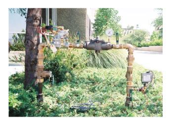
The BIC Station is a pre-engineered irrigation control valve station that incorporates a master valve, regulator valve, backflow preventer, preload valve and high pressure lock out switch in one "off the shelf" package. Installation is quick and simple, just drop-bolt-and go, since the whole station is above ground, no costly ground work is required.
