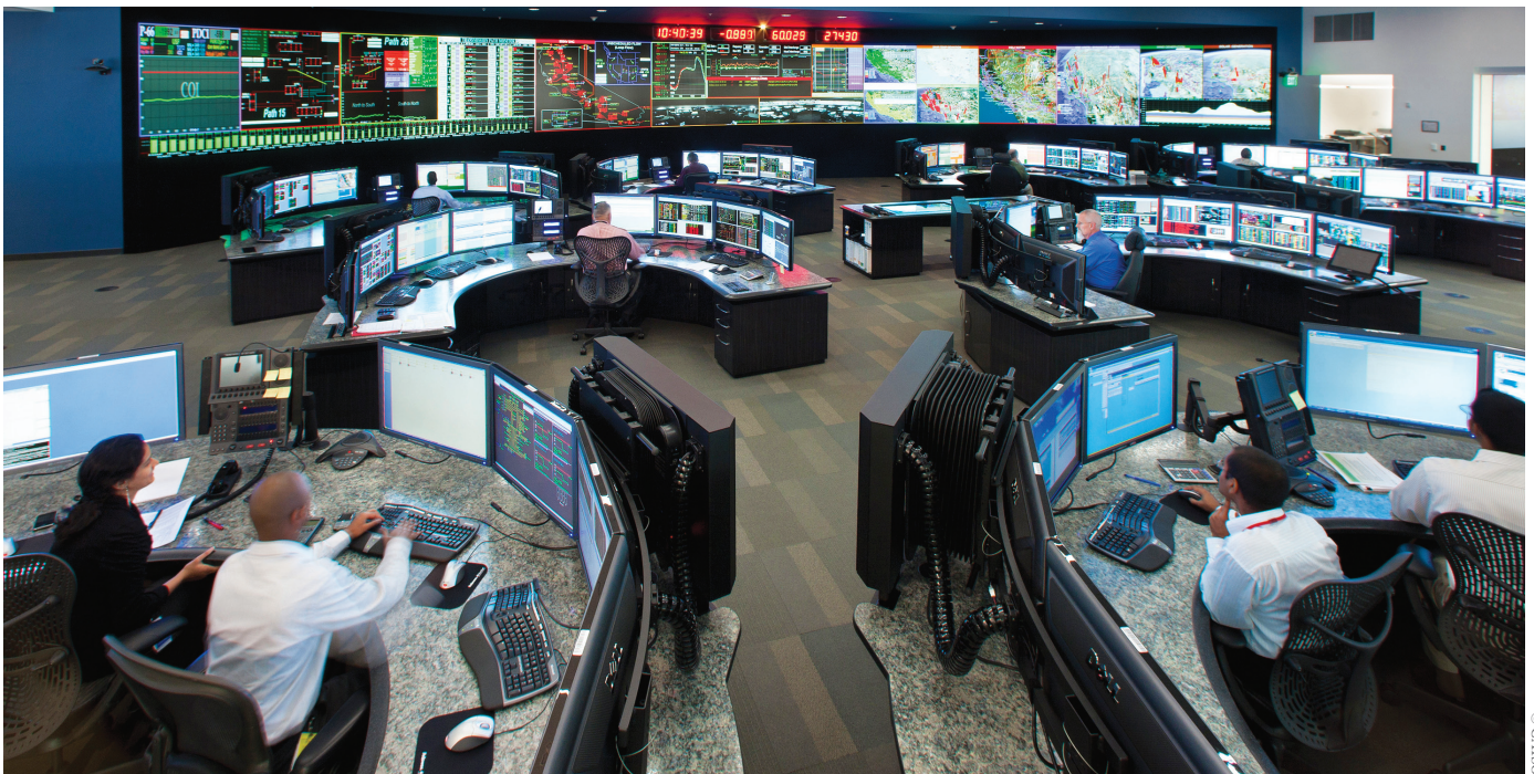
At the California Independent System Operator (CAISO) grid operation control center, electricity supply and demand are constantly balanced to maintain reliability.
