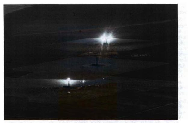
**Photo 2**. Photo of the ISEGS site taken from the north. From left to right: Tower 1; Tower 2, not in operation; and Tower 3. The photographer's position in relation to heliostat position and orientation results in no DSRH from Tower 1, but strong DSRH from Tower 3 which causes disability glare.
