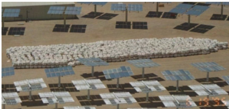
Figure L-1. 1.3 million kg (2.8 million pounds) of nitrate salt awaiting melting at Solar Two.
