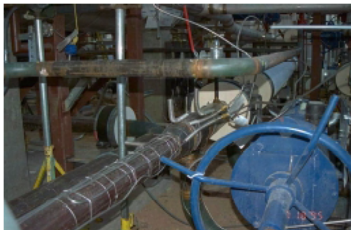
Figure Q-3. Multiple heat trace cables were applied to pipes that drained nightly to allow a two-hour heatup time the next morning. One or two spare cables were installed as well. A lesson learned was that heat trace must be installed uniformly (i.e. constant value of W/ft); otherwise, hot spots can occur that lead to pipe corrosion. A nonuniform section of heat trace is seen in this photo (see loop back). During the rework of the heat trace system in 1996, nonuniformities were eliminated.
