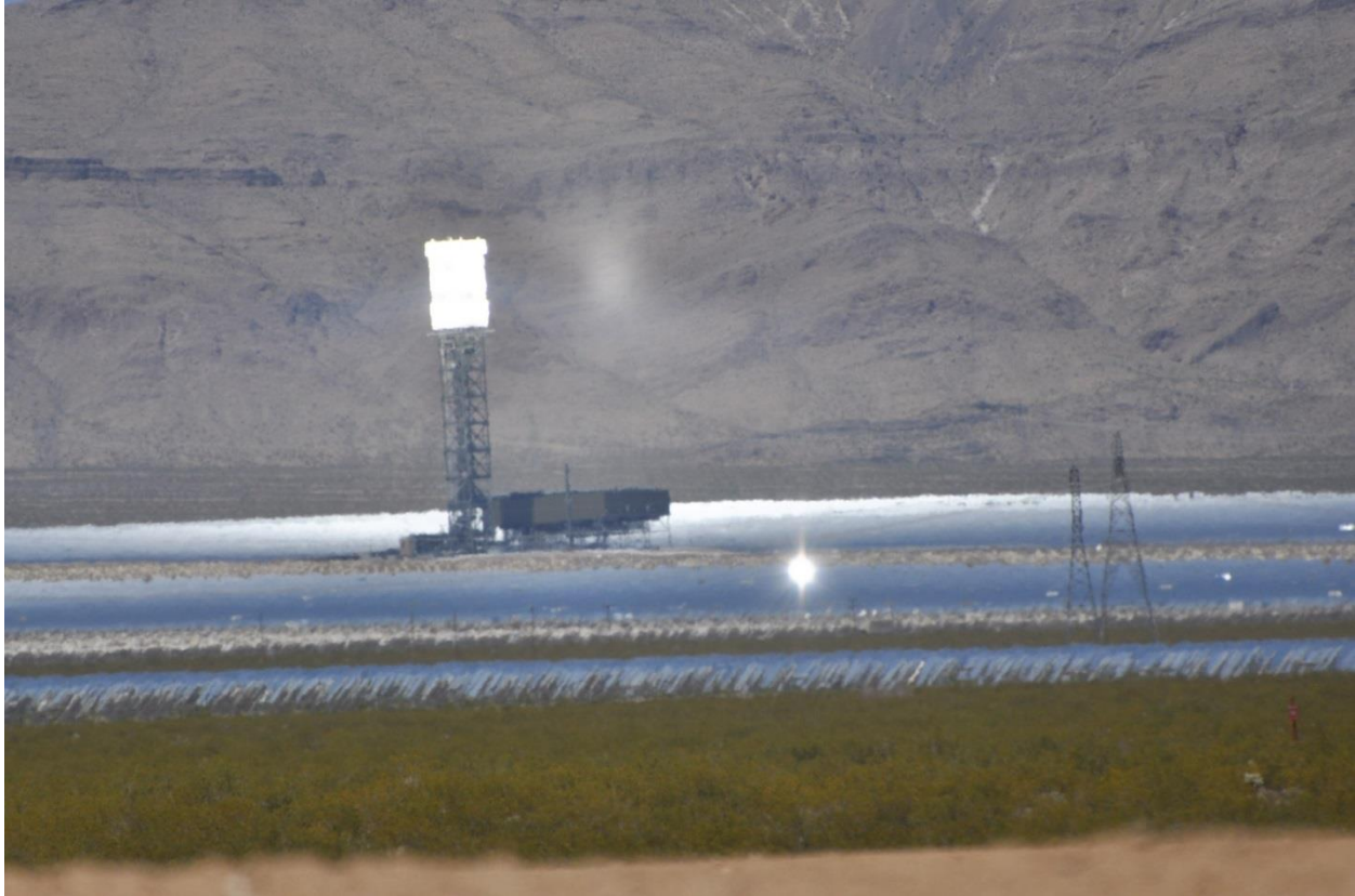
Figure 16. Photograph of Unit 3 receiver and “rogue” heliostat from I-15 (~3 miles away).
