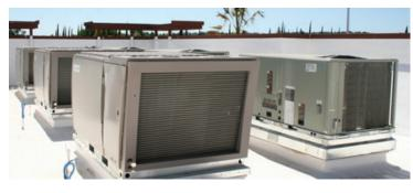
Figure 10 shows the Ice Bear storage commercial air conditioning unit. These devices actually provide both peak and energy savings, because they "make cold" at night, when temperatures are lower and the chilling units operate more efficiently, offsetting the usual "round-trip losses" associated with electrical energy storage.
