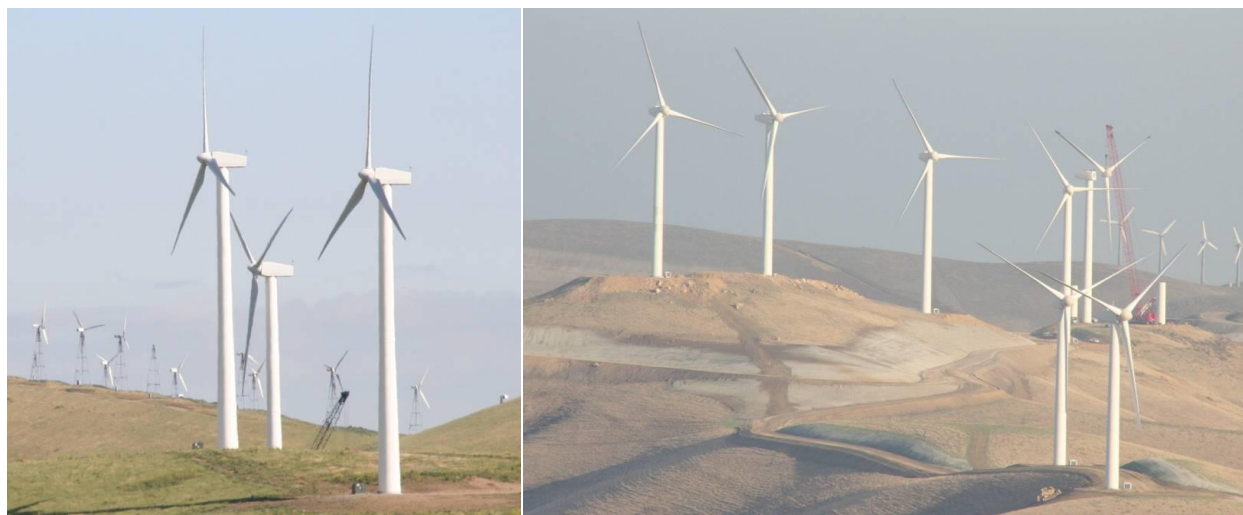
Figure 2. Vestas 660-kW turbines in Diablo Winds Energy Project, which replaced Flowind vertical axis turbines (left photo), and Mitsubishi 1-MW turbines in Buena Vista Wind Energy project that replaced Windmaster, Nordtank, and Danwin turbines (right photo).
