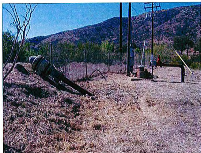
Photo 3: Pump Motor Assembly Removed and Placed by Well.
