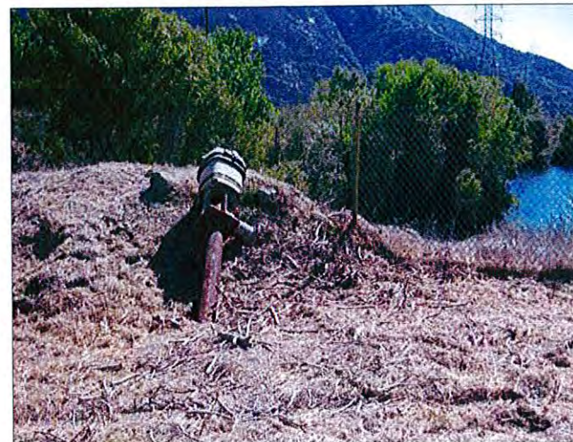
Photo 2: Pump Motor Assembly Removed and Placed by Well.
