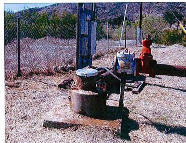
Photo 4: Locking Well Cap Installed.
