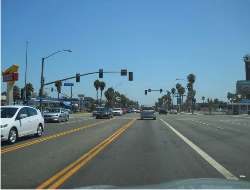
PCH to 2 nd Street
