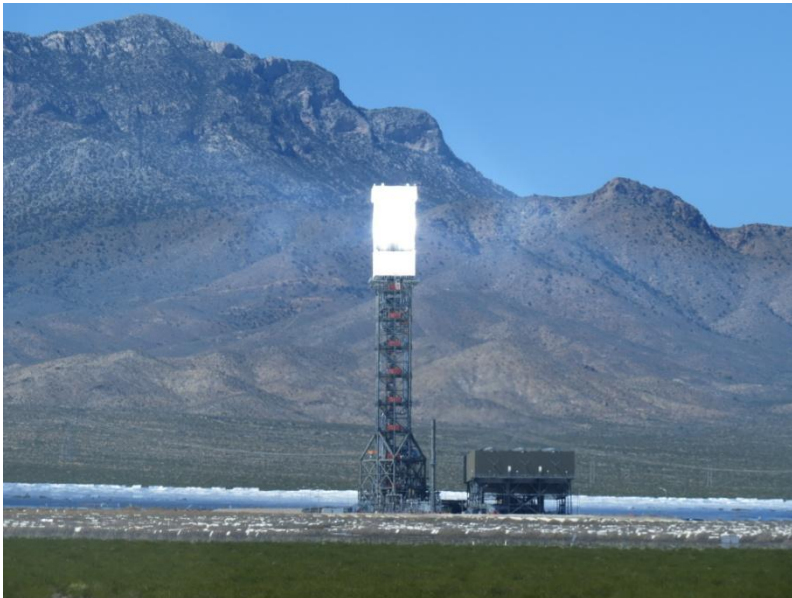
^Ivanpah Unit One being tested with Clark Mountain, Mojave National Preserve in the distance. Solar heat flux is highly visible, September, 2013
