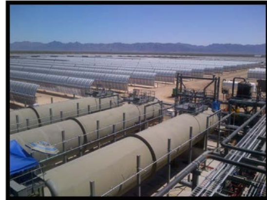
Power Block 1- Overflow Tanks
