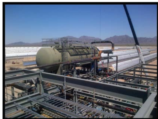
Power Block 1- HTF Expansion Tank
