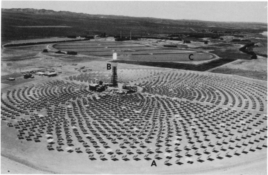
FIGURE 1. Aerial view of Solar One: (A) heliostat field, (B) central receiver tower, (C) evaporation ponds. Tower height = 86 m, diameter of field = 765 m.
