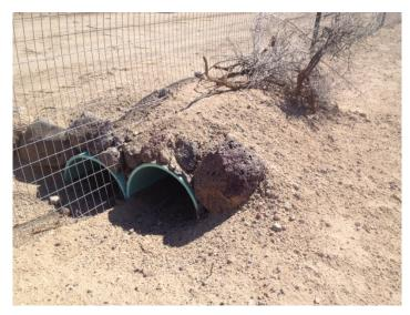
Figure 2: Desert Tortoise Shade Structure Installed along Rice Solar Energy Project Perimeter Fence
