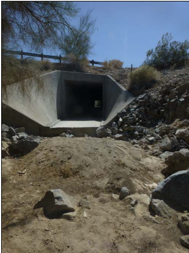
Photograph A-7. Box culvert I-10 underpass west of the modified gen-tie.
