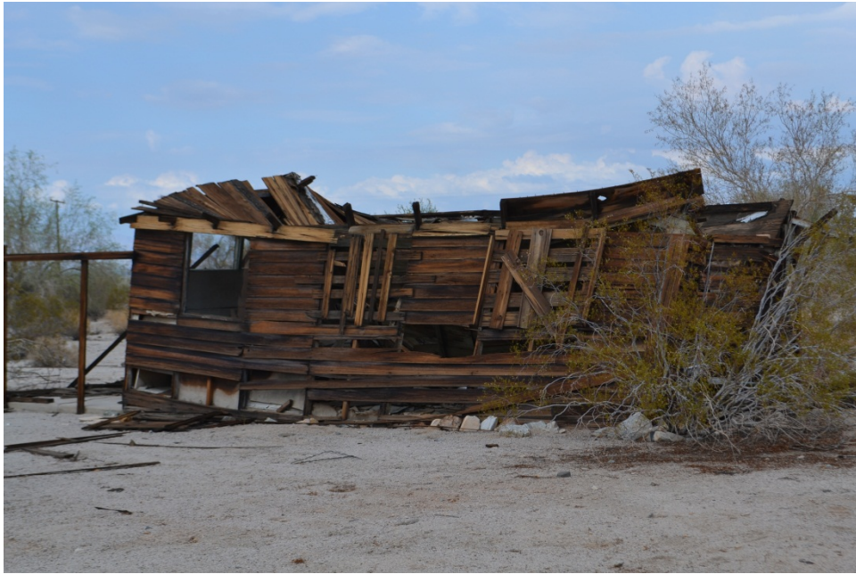
Photograph 10. "Shanty #10," Camera facing NE, DSC_0176, 7/11/13
