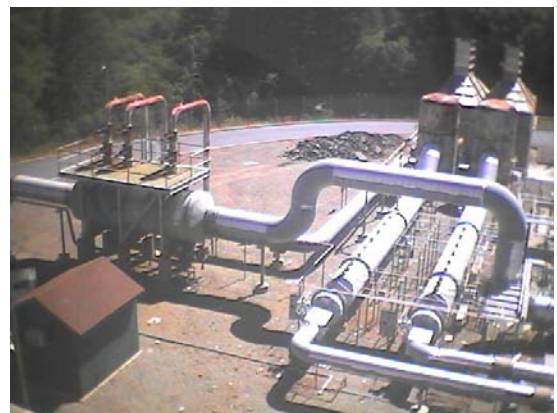
Steam Separator and Stacking System
